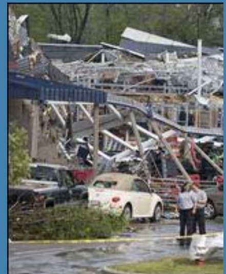
Sandford, Alabama - The Lowe's Home Improvement store, in Lee County, will re-open after it was destroyed by a tornado in April.
